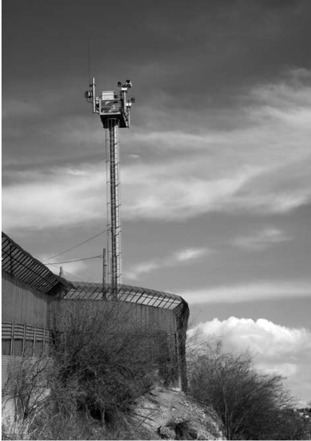
A surveillance tower on the U.S. side of the border fence, Nogales, Arizona
